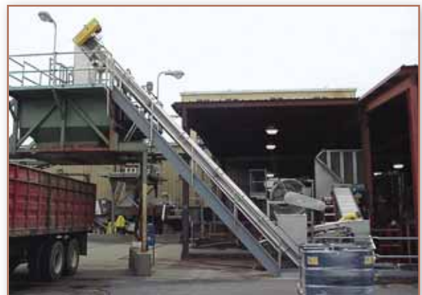
Installation of 24SWR.
